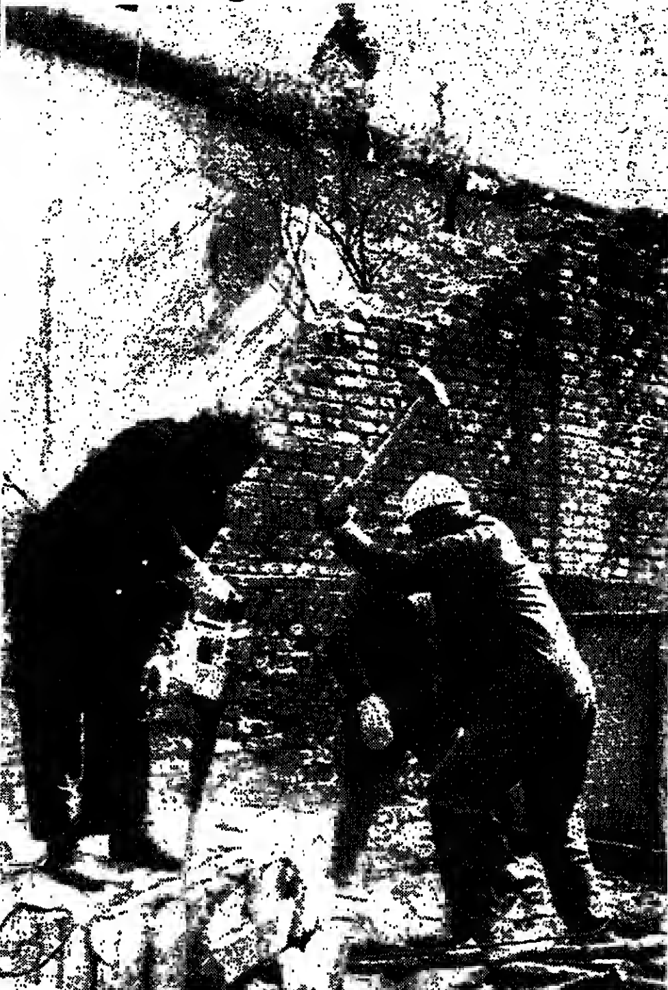
East Germans, working in West Berlin territory under the scrutiny of a border guard, remove stones of the old Berlin Wall, which broke down on Monday. Their watchful guard keeps his vigil from the new concrete wall. Meanwhile, early yesterday, two East Germans used a ladder to get over the Wall to the West because their applications to leave legally had been rejected.
